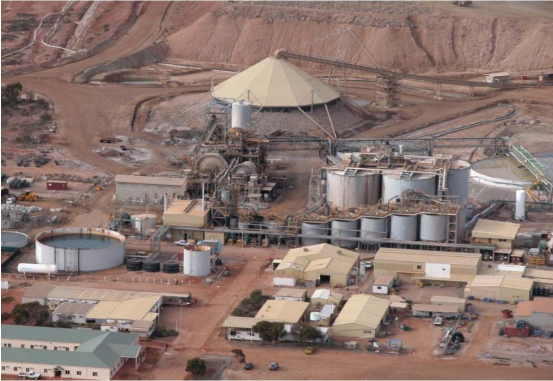
Paddington Processing Plant
