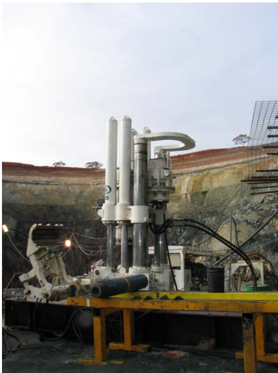
Raise boring a temporary return air way at Raleigh
