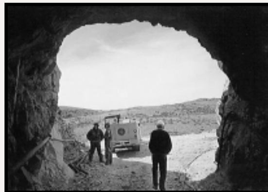
PORTAL OF THE MARTHA MINE DECLINE.
