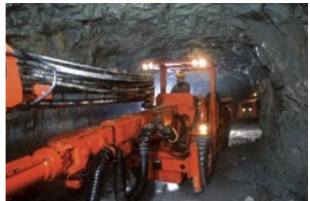
JUMBO DRILL AT THE MARTHA MINE.
