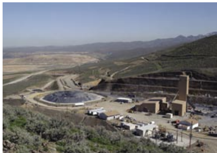
AERIAL VIEW OF THE WEST LEEVILLE OPERATION.
