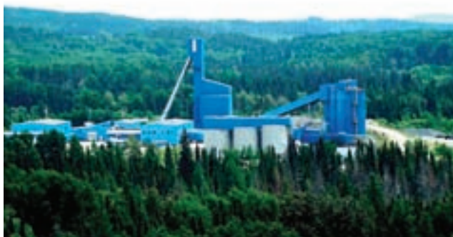
Holt mine site
