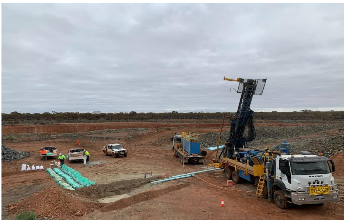
Fig 2. First drilling at the Paris Project – 25 June 2021
