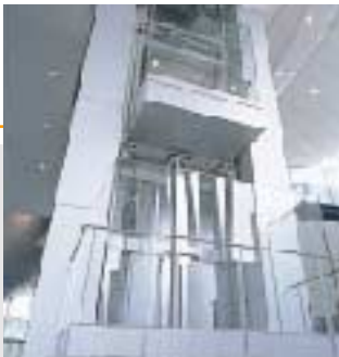
The panorama elevator at Saga Prefectural Aerospace Science Hall is an attraction in itself. It holds up to 43 people and travels at a speed of 35 meters per minute.
