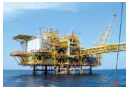
Ultra provides oilfield surveillance systems
