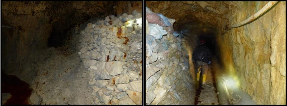
**Figure 5 – Cross-Cuts on the Siglo XX Level Adit Filled With Sludge, Mullock and Bagged Tailings**
