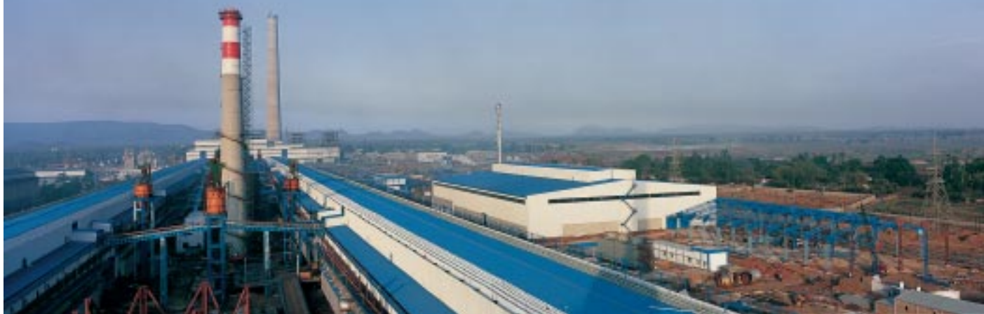
The two new pot rooms at Korba, each 1 kilometer long and containing 144 pots
