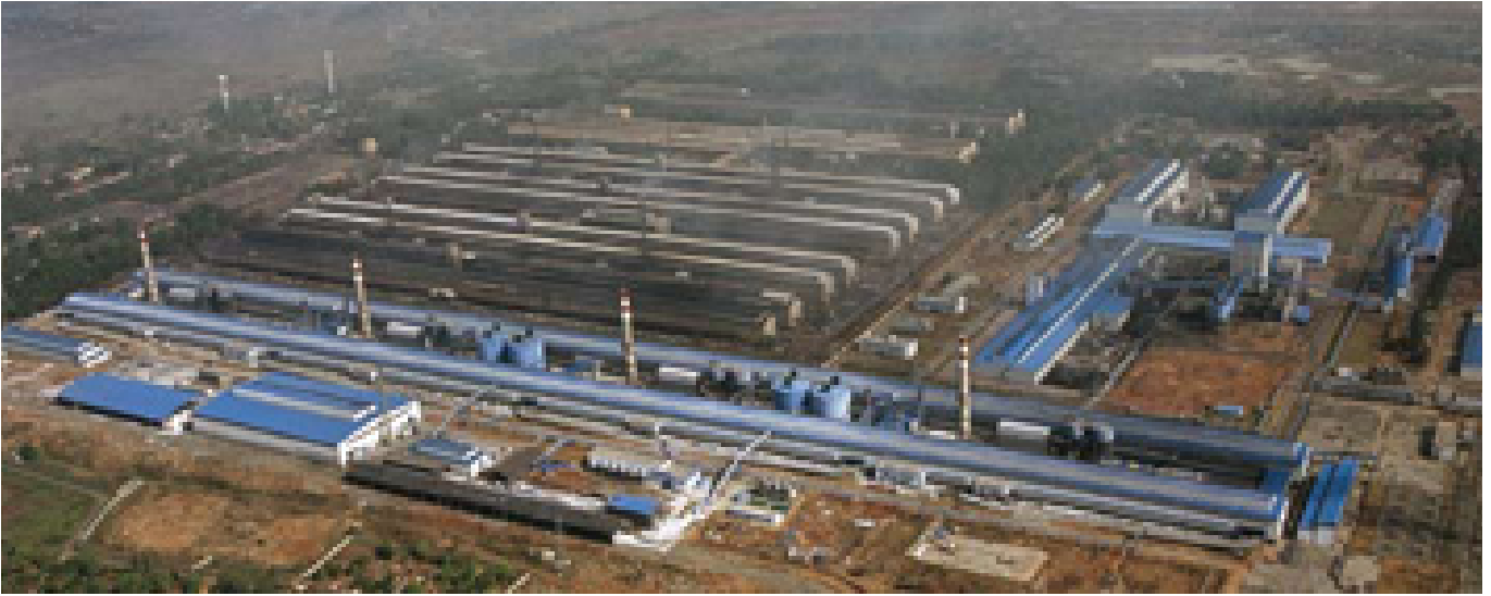
Aerial view of Korba II smelter
