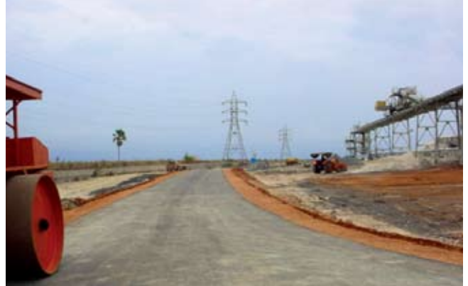
Road constructed from copper slag
