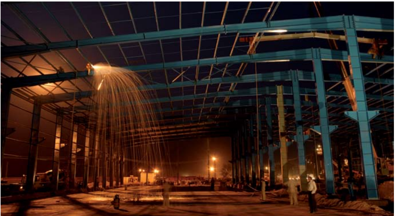
Work in progress at the Jharsuguda aluminium project
