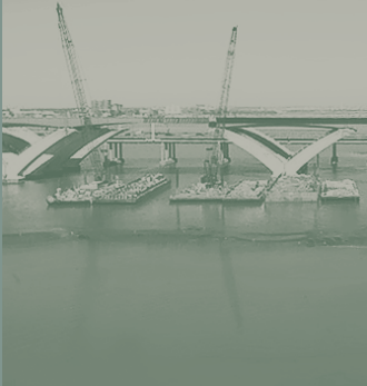
ALEXANDRIA, VA WOODROW WILSON BRIDGE PROJECT
