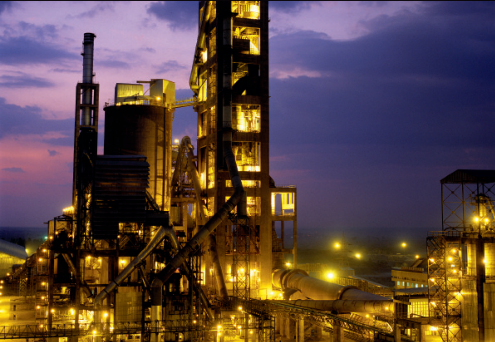
Cement factory where a number of RINGFEDER POWER TRANSMISSION's products are installed.
