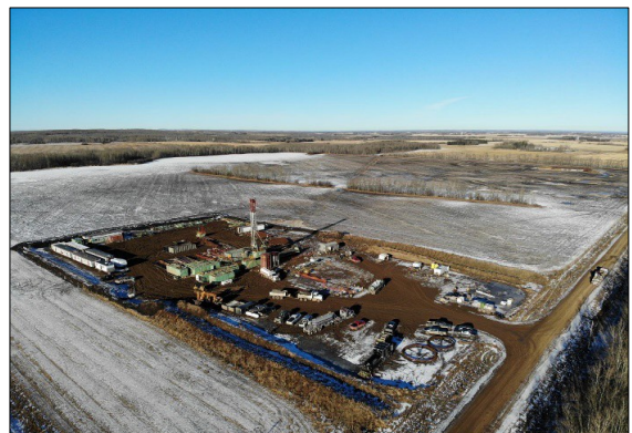
Figure 3 - Rex-3 during drilling
