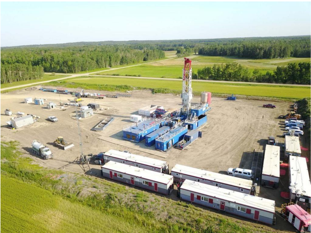
Figure 5 - Drill rig on site at Rex-4
