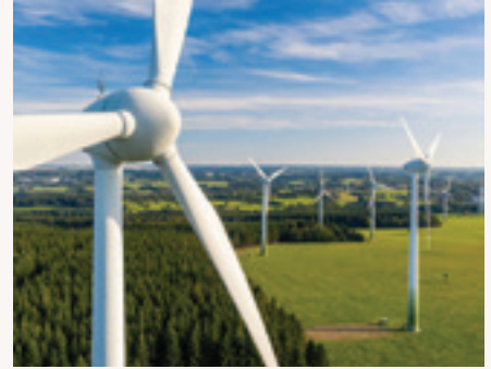
Wajax's ERS team has extensive experience in the maintenance and repair of wind turbines across Canada.
