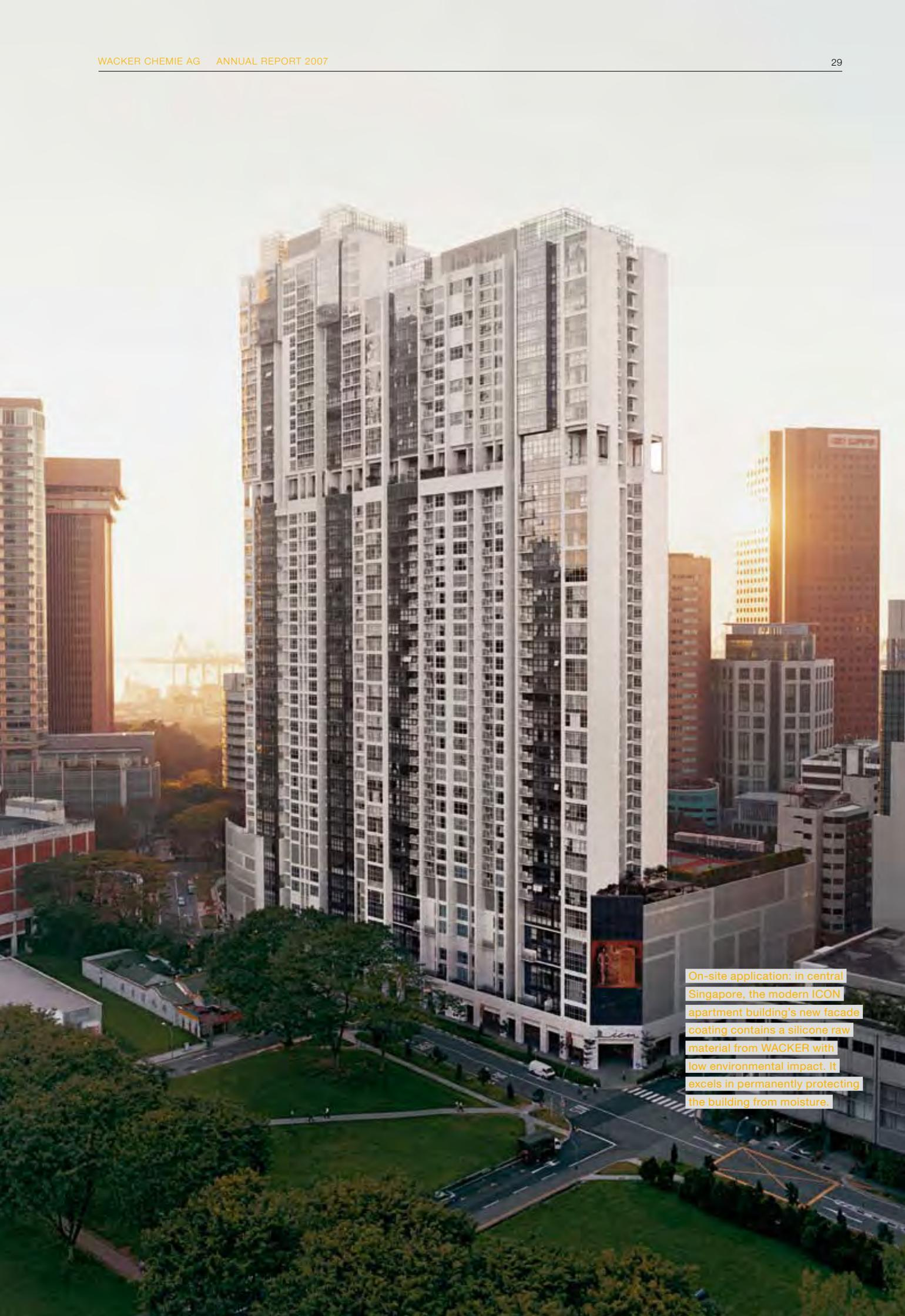
On-site application: in central Singapore, the modern ICON apartment building's new facade coating contains a silicone raw material from WACKER with low environmental impact. It excels in permanently protecting the building from moisture.
