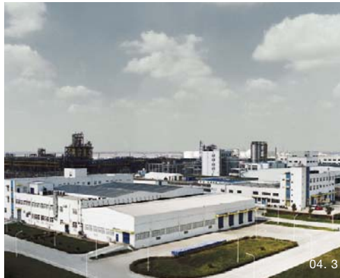
04. 3 The new WACKER site in Zhangjiagang.
